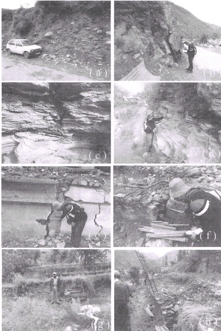
Figure 5: Subplot (a) Coarsely laminated fluvial deposit towards the crown of the landslide; (b, c, d) highly weathered schist and un-weathered gneiss with wide open fractures towards the crown of the landslide; (e & f) cracks developed in the concrete structures; (g) landslide scar developed within the slide mass; (h) tilted retaining and longitudinal landslide scar.
